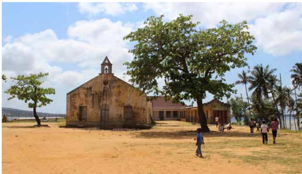
A view of Maxixe during an on-site visit, courtesy of DASTU.
